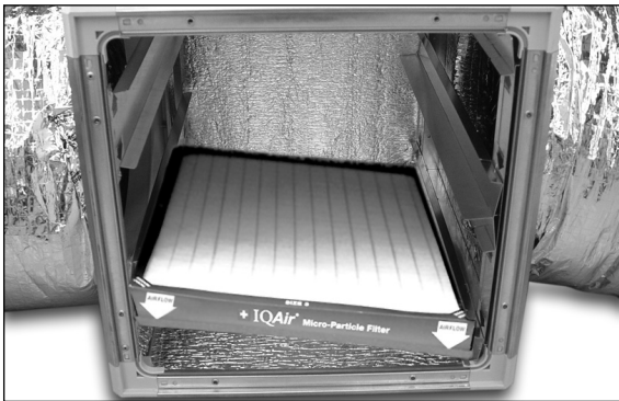
5. Insert new filters starting from the bottom.
