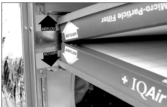
6. Ensure that you align the filters with the airflow arrows matching the airflow arrows on the cabinet.
