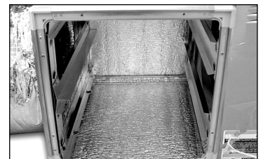
6. Remove filters and secure via panel from inside to the air handler.
